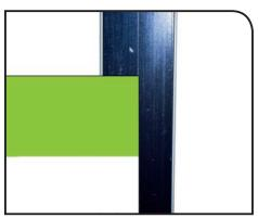
• Check the graphic panels are lined up with the centre line of the magnetic bar, if this overlaps by just a little it will give the appearance that part of the magnetic bar will not work
